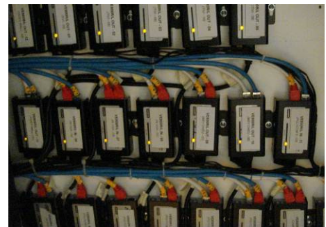
ATEN HDMI Extenders uses Cat 5e cable to extend the distance between source and display devices
