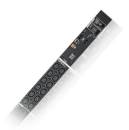
As part of its NRGence line, ATEN has developed a new generation of green energy power distribution units (eco PDUs) to effectively increase the efficiency of data center power usage. The NRGence PE7214 eco PDUs are intelligent PDUs that contain 14 AC outlets and are available in various IEC socket configurations.
